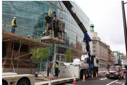
Refurbished statue being craned into place
