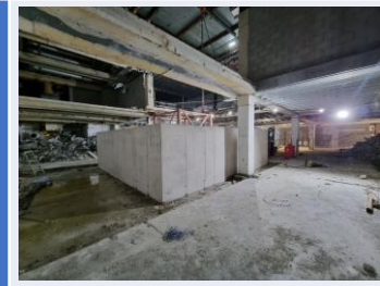
Tower crane base installation
