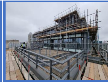
Upper terrace scaffold erection
