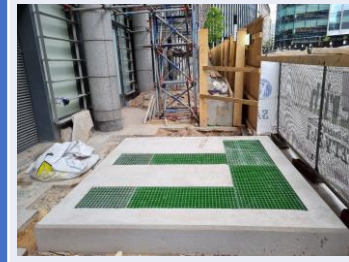
Temporary substation base
