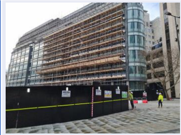
Saint Bride Street Scaffold erection
