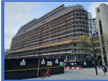
Completion scaffold on Saint Bride Street
