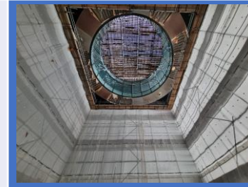
Internal atrium scaffold
