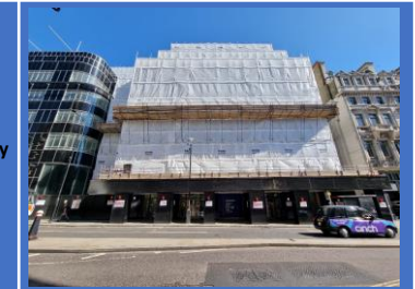
Fleet Street hoarding & scaffold erection
