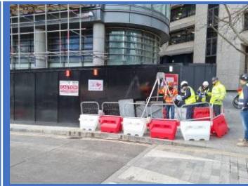
Dilapidation Survey to CoL Tunnel
