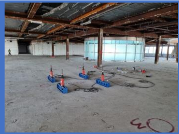
Floor Load Testing
