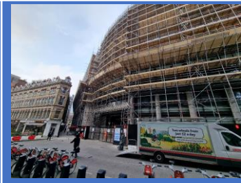
Poppins Court scaffold and loading bay
